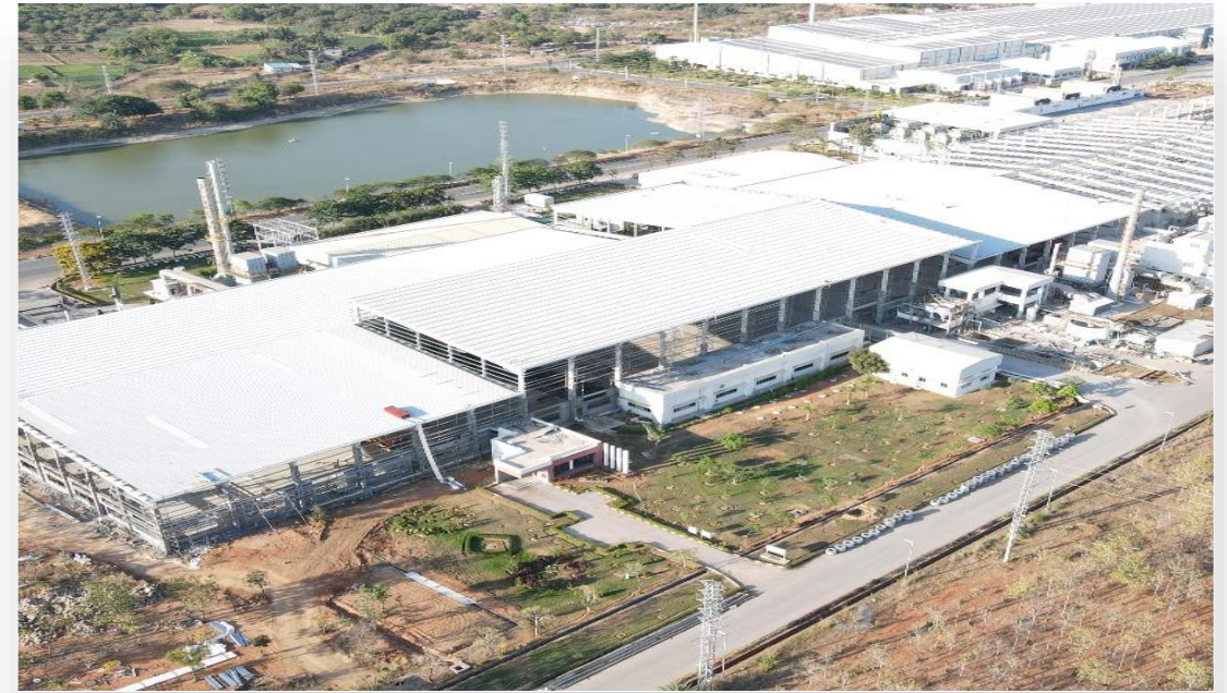
Tubular Battery Plant at ARGC- Chittoor
